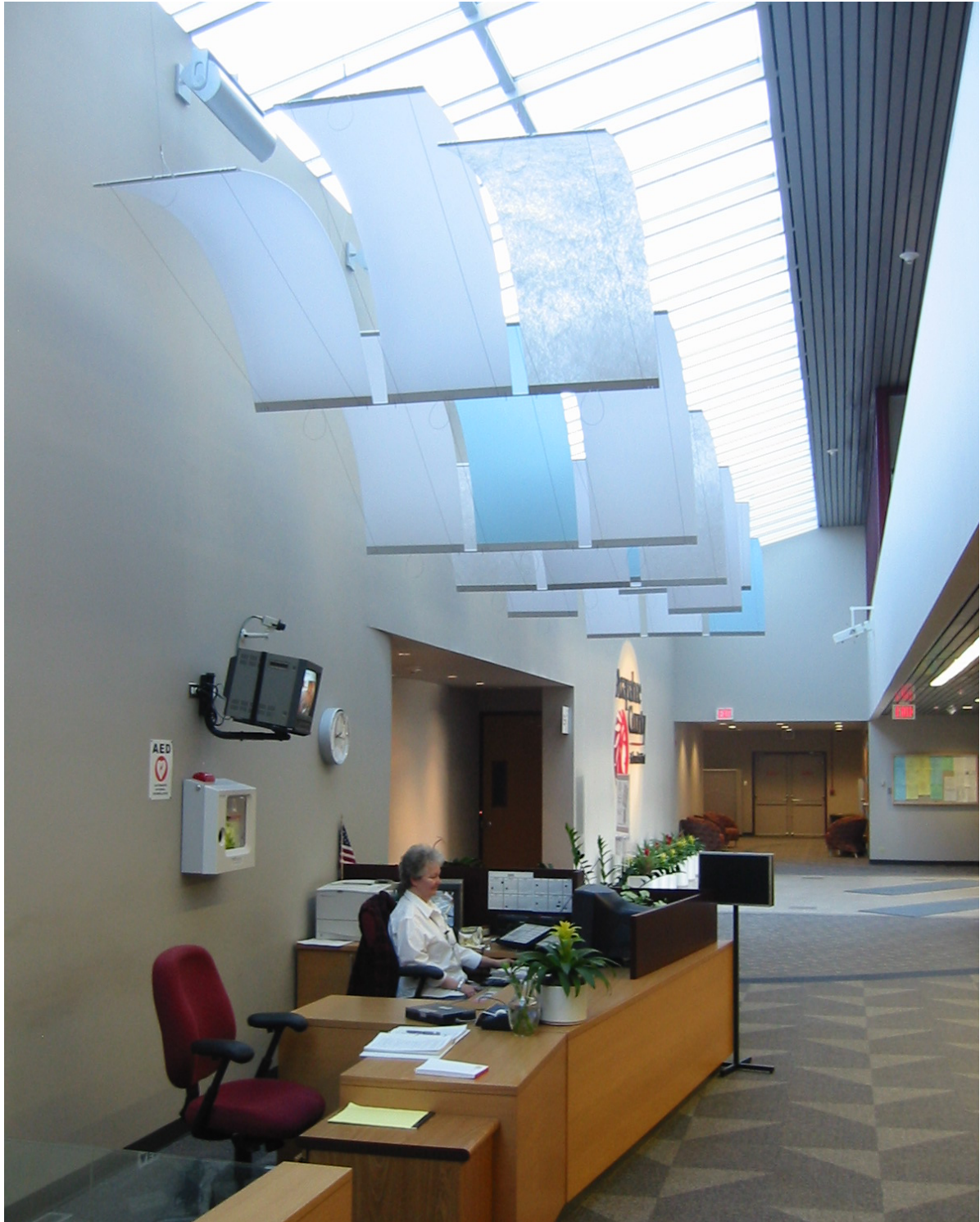
Skylight shading system using Armstrong suspended acrylic panels, reducing the intensity of the skylights and redirecting the light onto the ceiling, eliminating glare.
