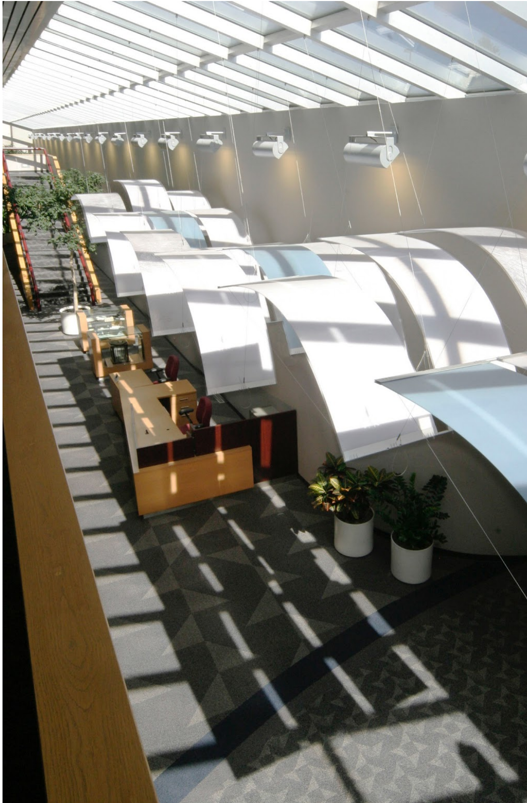
Skylight shading system using Armstrong suspended acrylic panels, reducing the intensity of the skylights and redirecting the light onto the ceiling, eliminating glare.
