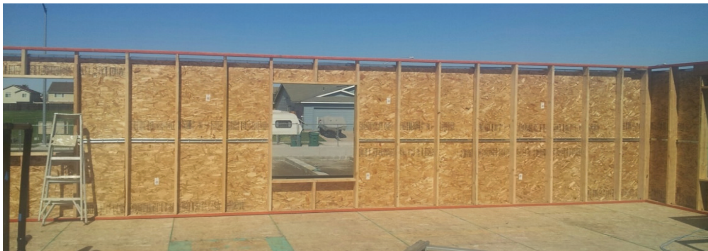
Example of window placement in advanced framed wall
